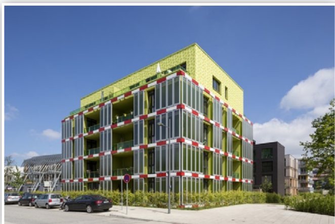
The "Algae House," a project of the IBA Hamburg, is a passive energy building with a bioreactor façade
