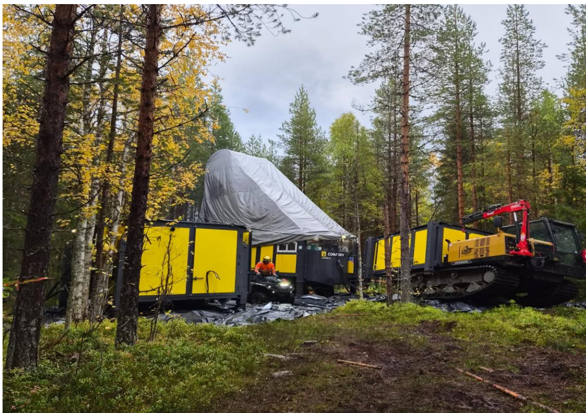
Figure 1 - Drill rig establishment at the Central zone
