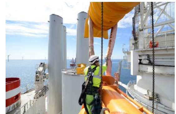
Leading installation company with ~900 employees
