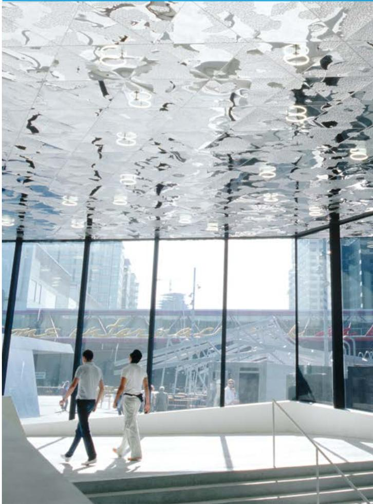
In the architectural masterpiece Edificio Forum in Barcelona, Spain, 28,000 panels of Outokumpu Supra austenitic stainless steel create a finish that replicates the surface of water.
