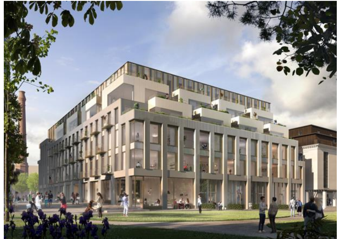
Veidekke is building Mineralvandsfabrikken in central Copenhagen and will contain commercial and residential units
