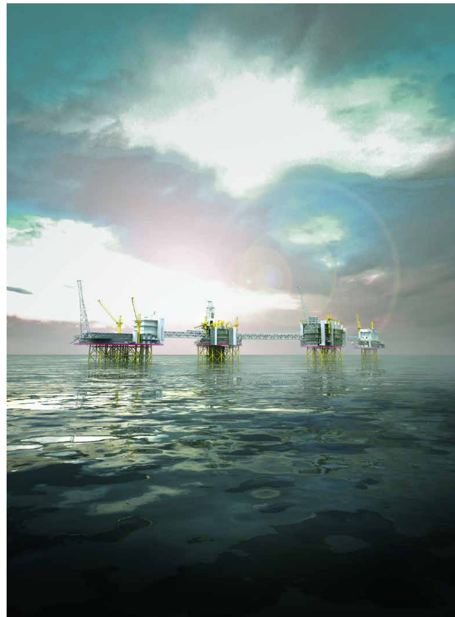
Development concept: The field centre will, in the first phase, consist of a processing platform, drilling platform, riser platform and living quarters, and has been designed so as to facilitate capacity for future development. Illustration: Statoil
