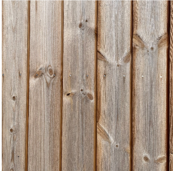
Figure 25: Boards with higher sapwood ratio on the external surface to the left and with higher heartwood ratio on the right. Picture from building where Material B was collected.
