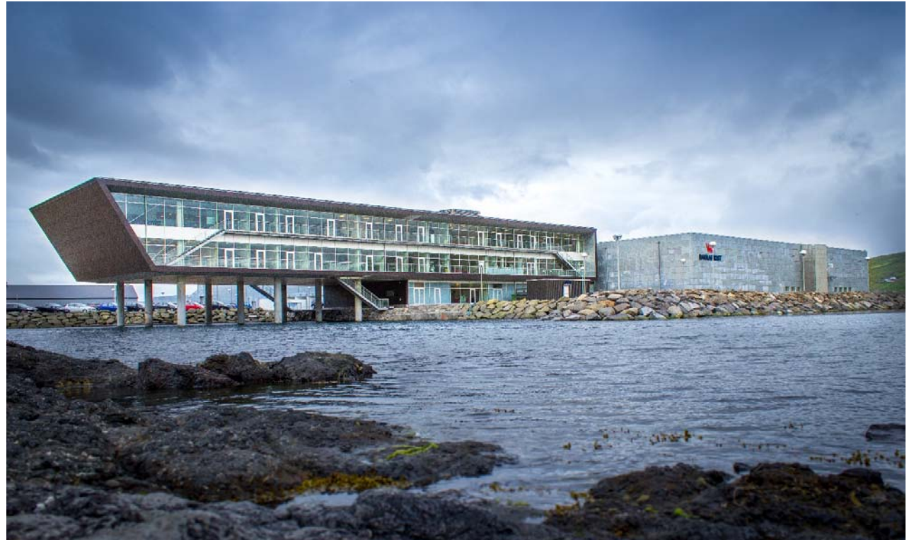
Bakkafrost HQ Glyvur
