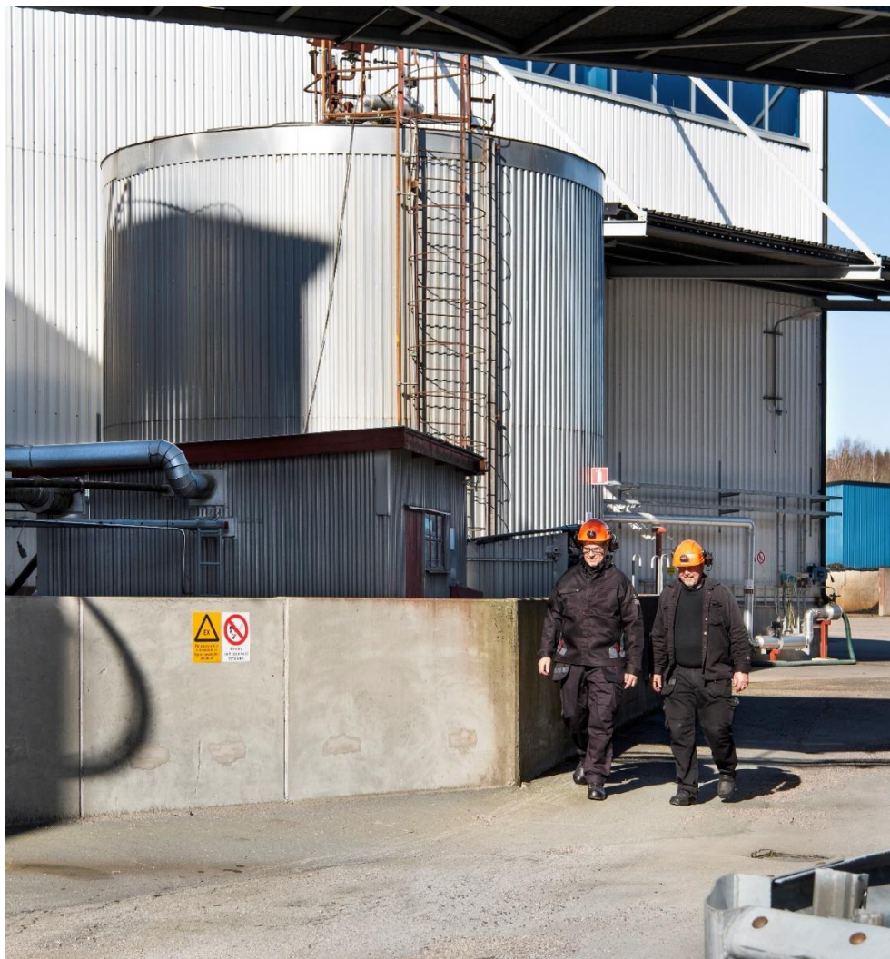
In the background you can see the tank where the Tyre Pyrolysis Oil (TPO) is being kept before dispatch from the plant in Åsensbruk. With the current mix of End-of-Life-Tyres this oil has a bio-content of approximately 48%.
