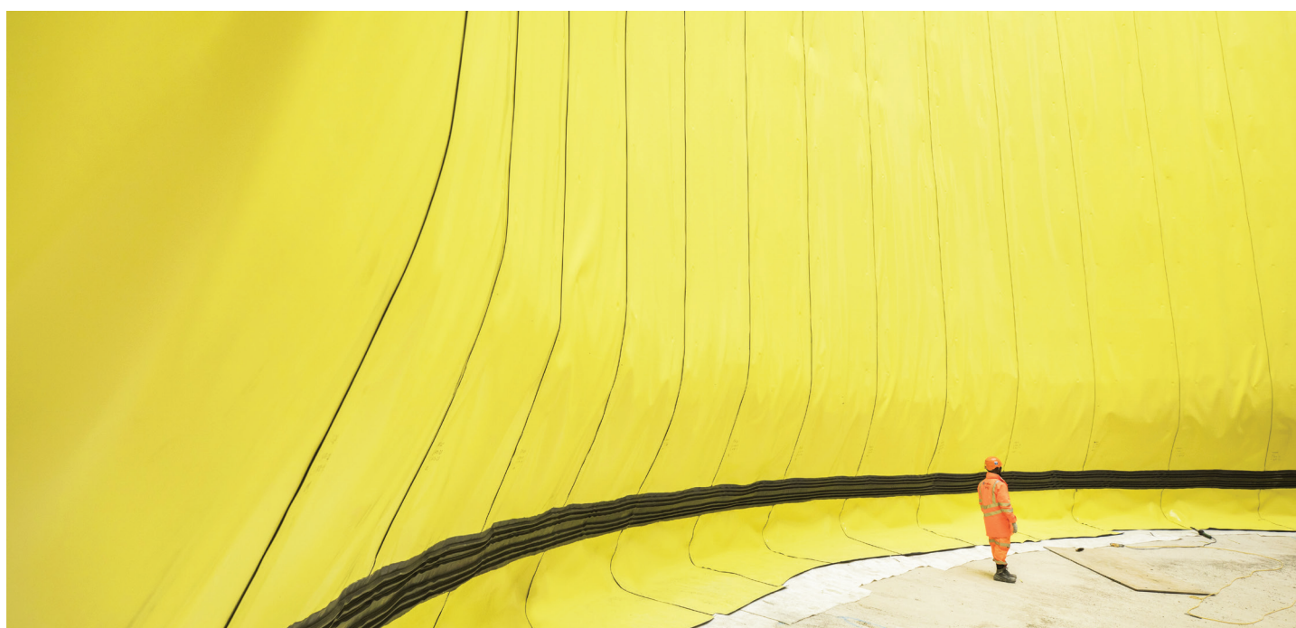
High Speed 2, Central Victoria Road, London, United Kingdom
