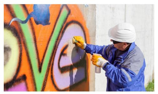
The new anti-graffiti coating from WACKER offers a fast, cost-effective means of removing graffiti. (Photo: Wacker Chemie AG)
