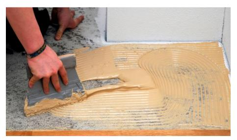
One of the products that WACKER will be presenting at ABRAFATI is GENIOSIL® XM 20, an alpha-silane-terminated polyether that yields plasticizer-free adhesives with exceptionally high elasticity. Typical applications include wood-flooring adhesives and allround adhesive sealants (photo: Wacker Chemie AG).
