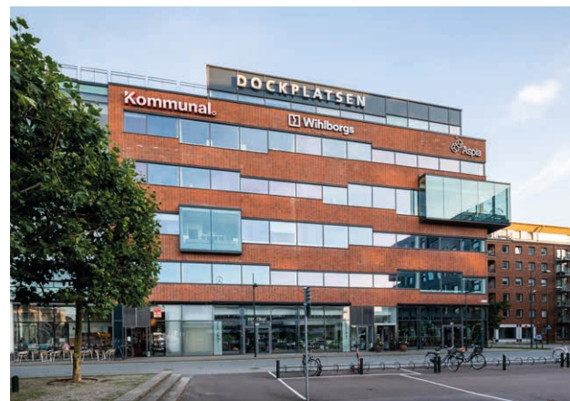
At Skrovet 3, home to Wihlborgs’ headquarters among other tenants, operational optimisation measures have resulted in a 33 per cent reduction in energy consumption.
