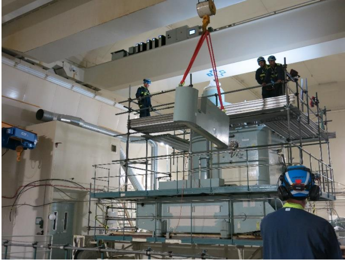
Nedmontering. Foto Rodrigo Prieto
