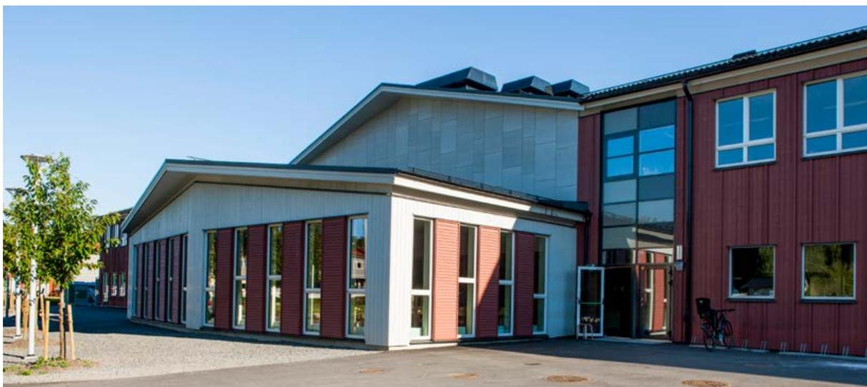
**Vendelsö 3:1986** Vendelsö is a passive building that is heated by sun, internal heat gains and recycled heat in ventilation systems
