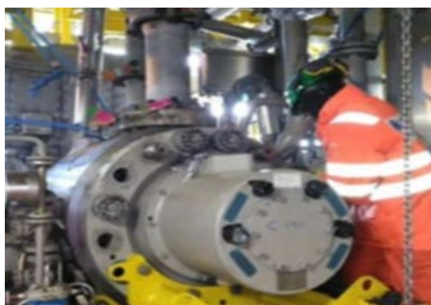
TEG export compressor bundle installation
