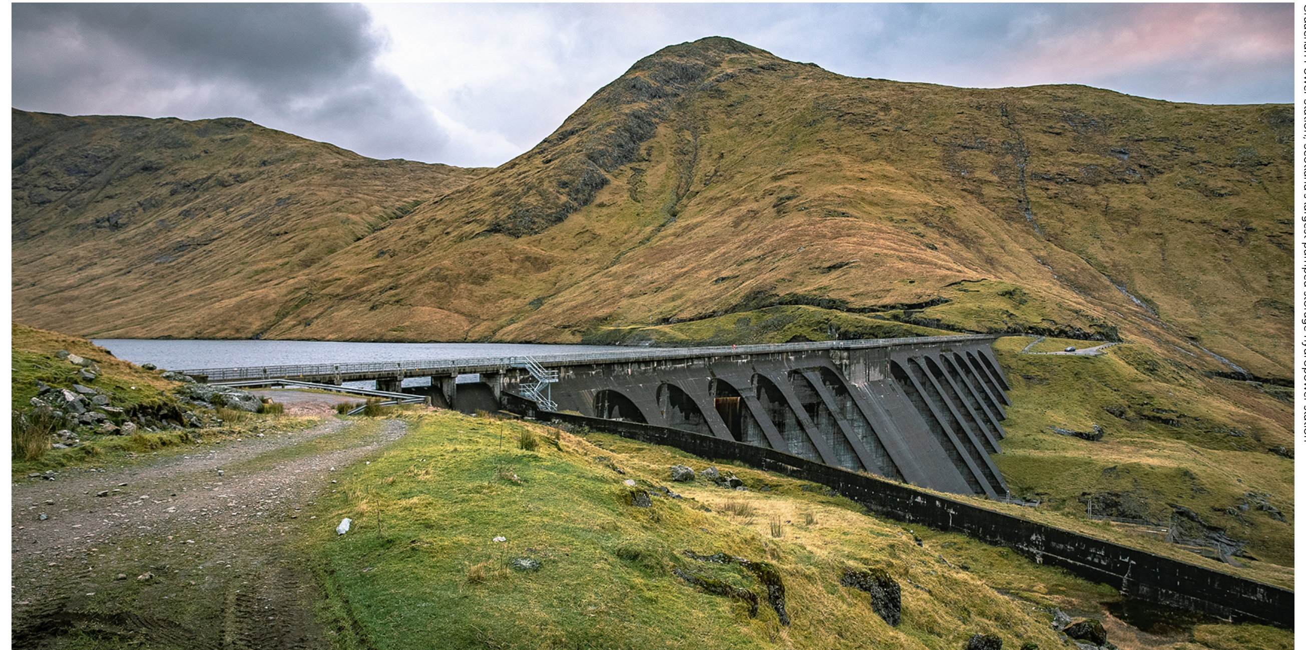
Cruachan Power Station, Scotland's largest pumped storage hydropower station
