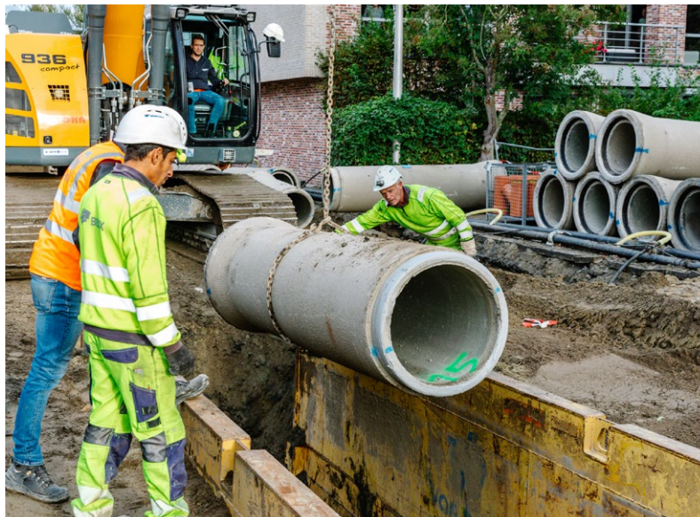
In Belgium, Tubobel builds a water system low-carbon pipes made with Betolar's Design mixes.
