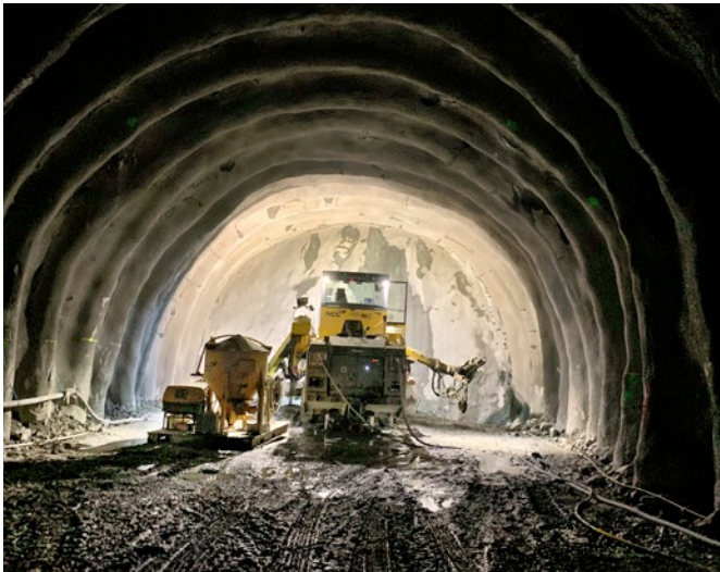
Blasting work in one of the tunnels at Breivika.
