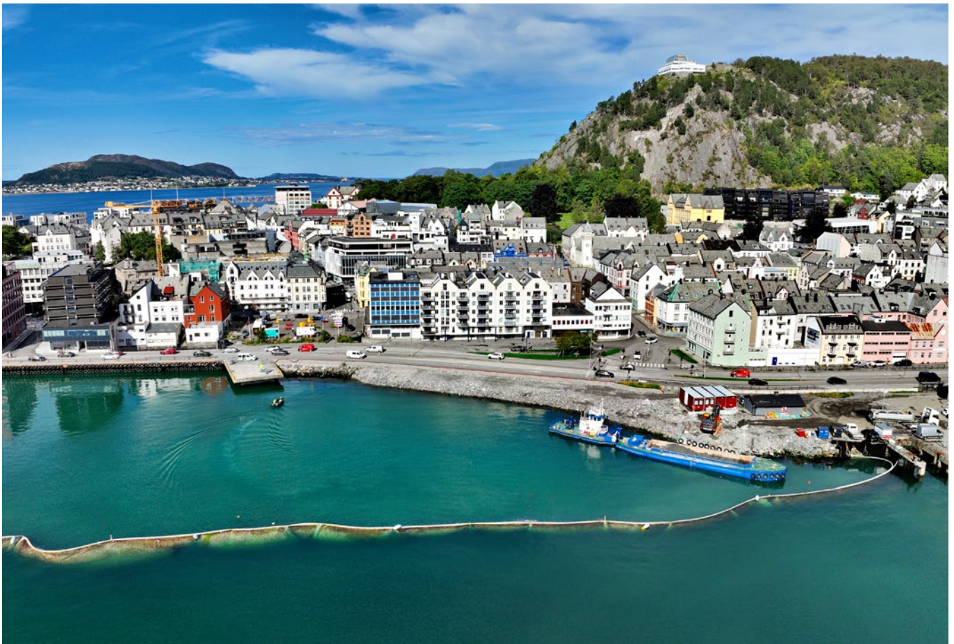
Landfill work in the Port of Ålesund.
