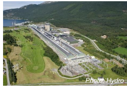
Husnes aluminium: Upgrade onshore plant
