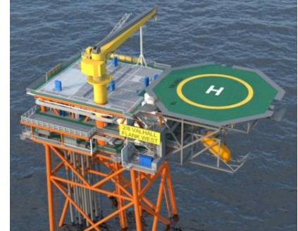
Valhall Flank West normally unmanned WHP
