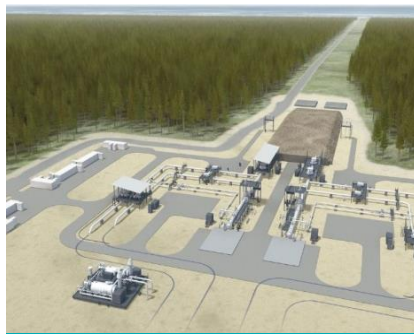
Nord Stream 2 onshore facility
