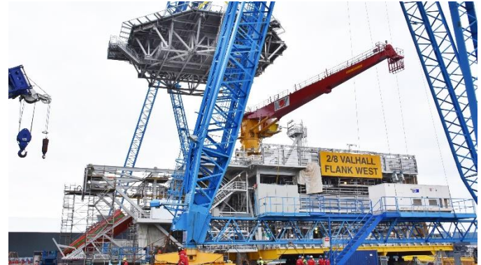
Valhall Flank Vest topside and jacket project
