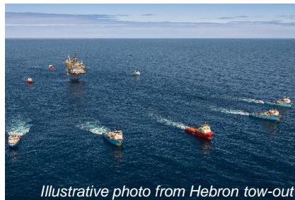
Marine operations for platform removal, Canada
