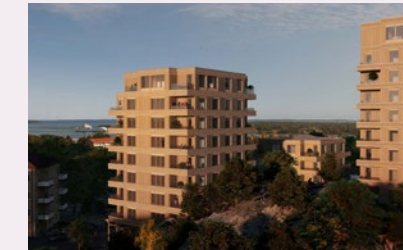
PANORAMA External contracting project
