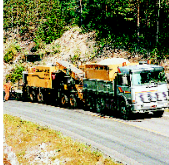
Microsurfacing Norwegian roads.
