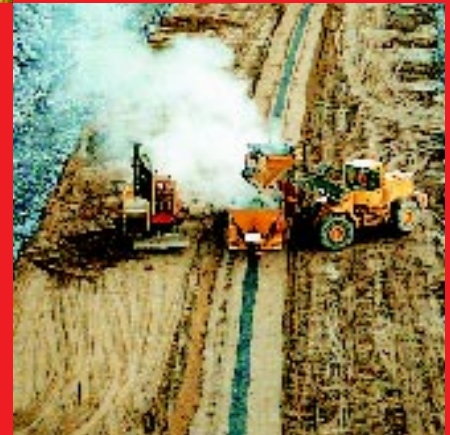
Veidekke/Korsbrekke og Lorck is the only Norwegian company with special knowledge of asphaltic cores in rock-fill dams. This technology has attracted a great deal of interest at home and abroad. Work of this kind is currently being carried out at Svartisen for Statkraft Anlegg as.
