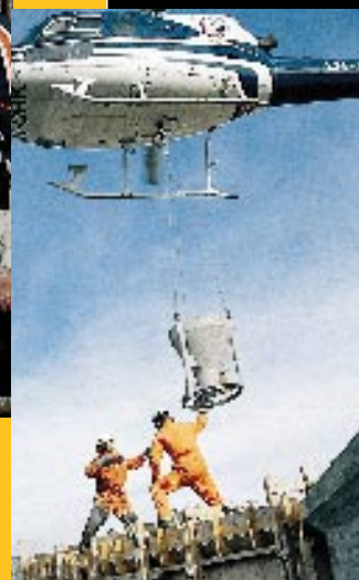
Veidekke project manager Anders Grimnes flies the helicopter. Jostein Myrann and Terje Leer guide the concrete skip into place for the last casting at the Reinevatn Dam in the Urar development in the Setesdal mountains.
