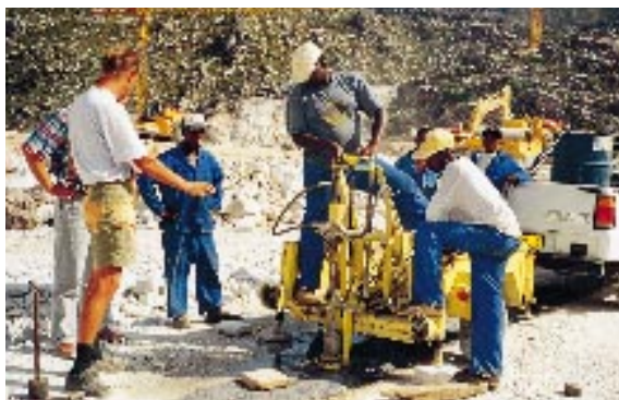
Ceres Dam near Cape Town in South Africa is the first rock-fill dam in Africa constructed with an asphaltic watertight core. Vermund Bjerkhagen is in charge of the work to remove a core sample to check that the 50-centimetre thick asphalt wall is watertight.
