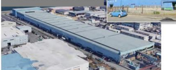
EXTERIOR VIEW OF FACTORY BUILDING
