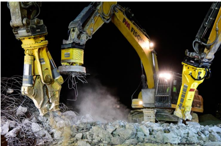
From left: A hydraulic cutter, magnet and breaker, each attached to an excavator, are some of Epiroc's hydraulic attachment tools.
