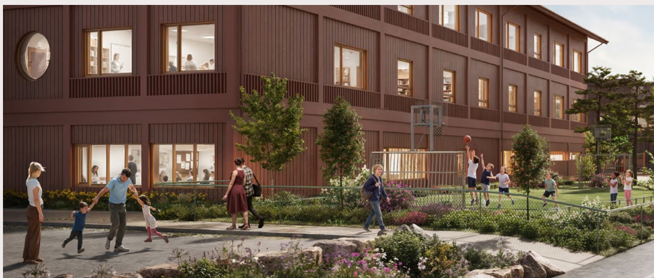
The Raoul Wallenberg School is being constructed in wood, with red wood panelling.
