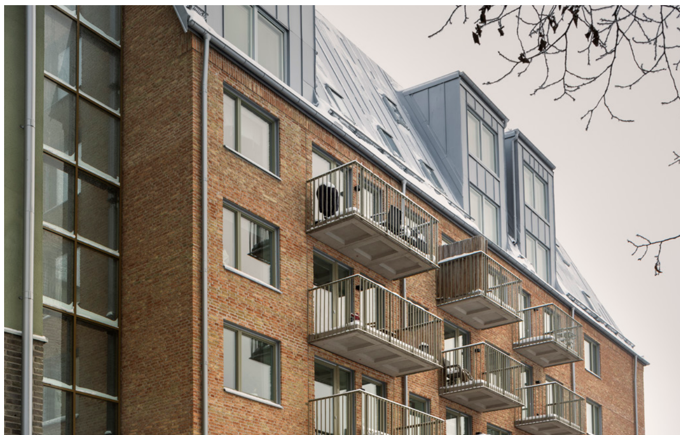
The Segerdal project is located in central Knivsta, directly adjacent to the train station. The first block has been completed and tenants have moved in. The second block, which is under construction and to be completed in November 2025, contains 151 rental apartments. The project is being carried out in a joint venture with Redito.
