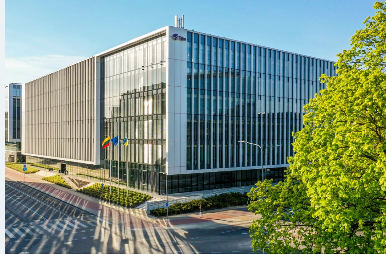
In the central business district in Vilnius Eastnine owns, among other, property S7-2 with Telia as tenant.
