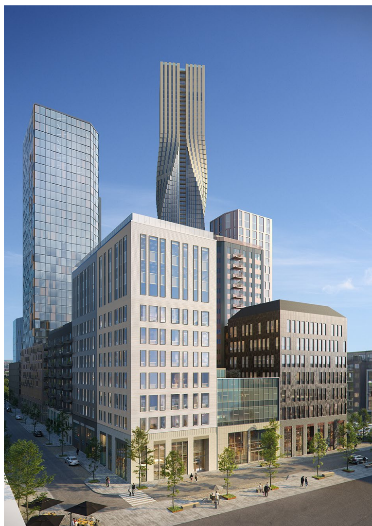
The Capella neighborhood is starting to grow in Karlstad in collaboration with Hemsö and Tosito. In addition to housing, premises for care, education and care will be housed in the neighborhood.
