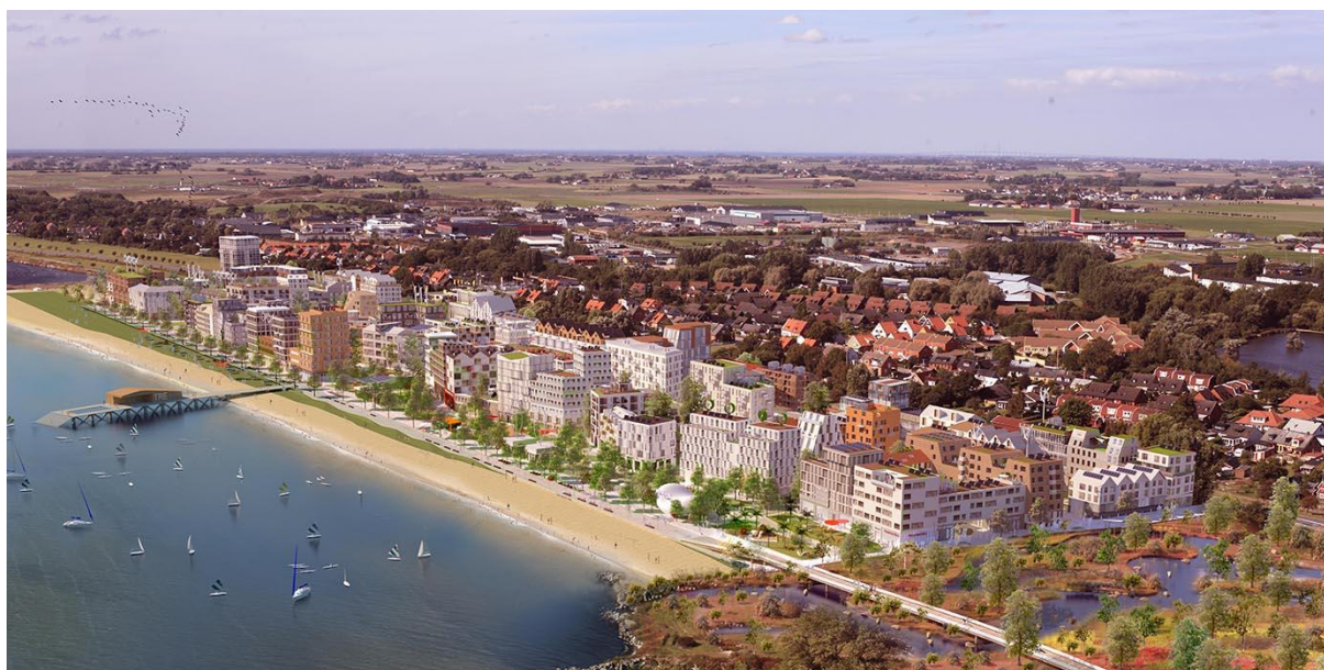
Serneke and Midroc have signed a letter of intent with the Municipality of Trelleborg regarding the development of a new district in central Trelleborg. Västra Sjöstaden, the project's working name, is part of Kuststad 2025, Trelleborg's major urban development project.
