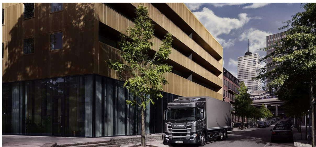
Serneke Construction has signed an agreement with Scania Industrial Maintenance to construct a new office building for 425 people in Södertälje. The contract also includes an option to construct another office building of an equivalent size.
