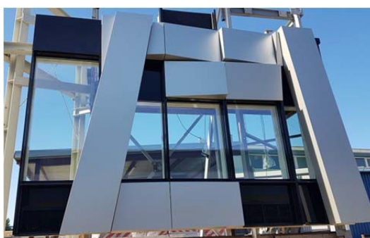
A demonstration of the façade element at Staticus production site in Lithuania
