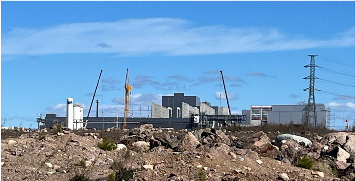
Figure 4: Easpring cathode plant in Keltakallio site
