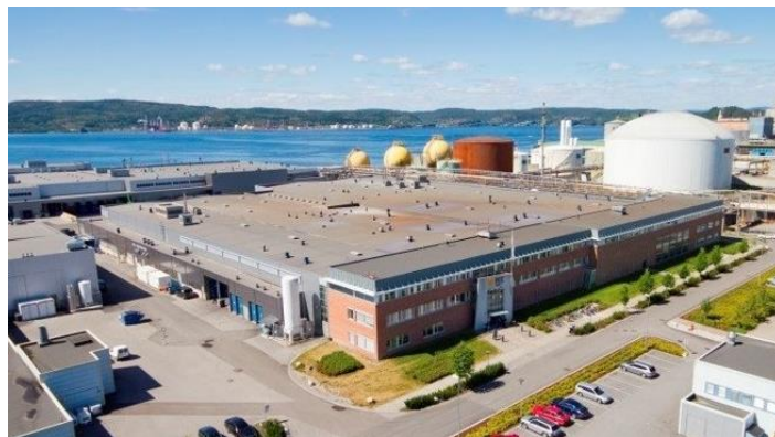
The secured premises at Herøya Industrial Park has an area of 15,000 m 2
