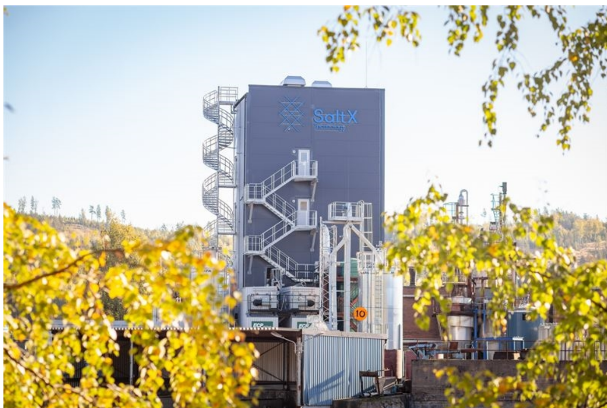
Photo: SaltX facility in Hofors, Sweden.
