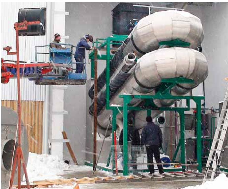
The flue gas condenser at the sawmill and combined heat and power plant in Olczyk, Poland, was assembled during harsh winter conditions. The condenser now produces up to 4.9 MW of heat.
