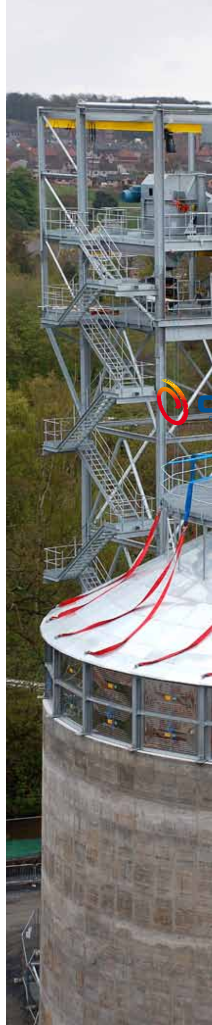
The roof of the first of the three silos that Saxlund is building is lifted into position late in the evening. This is a part of the bioenergy plant that energy giant RWE npower renewables is installing for paper maker Tullis Russell in Fife, Scotland.
