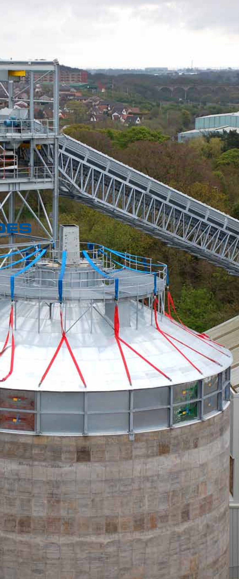
Each 26-m tall silo can contain up to 5,000 square metres of woodchips and is equipped with Saxlund's rotating TubeFeeder®, which will convey the woodchips from the silos into the combustion plant.
