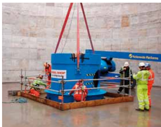
The roof of the first of the three silos that Saxlund is building is lifted into position late in the evening. This is a part of the bioenergy plant that energy giant RWE npower renewables is installing for paper maker Tullis Russell in Fife, Scotland.
