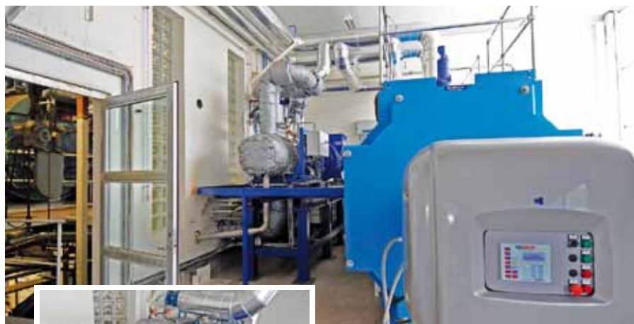
P o B Energi was able to place its Opcon Powerbox between a wall and the existing boiler.
