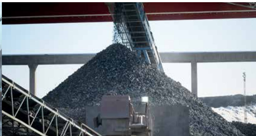
The iron ore is crushed in the industrial area and transported by conveyor into the sorting plant.
