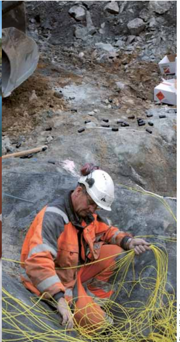
Preparation for blasting the shaft from the surface.
