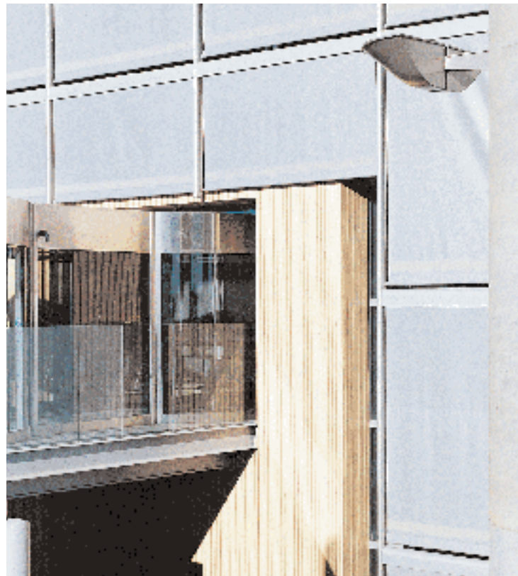
HMF impregnated (heavy metal free) external pine panelling – Oslo Airport Gardermoen.
