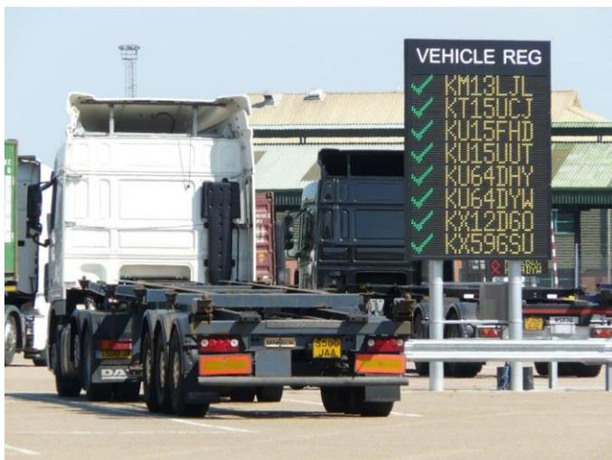
Installed in the trailer holding area, the bright and highly visible signs display the vehicle registrations of vehicles in the queue accompanied by a green tick or a red cross, so that each driver can see clearly when it is safe to proceed to their loading or unloading destination. Special attention to protection was paid when designing the signs, which operate within a harsh marine environment.
