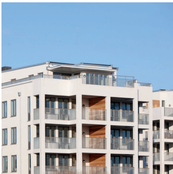
Victoria Park Brf Allén
